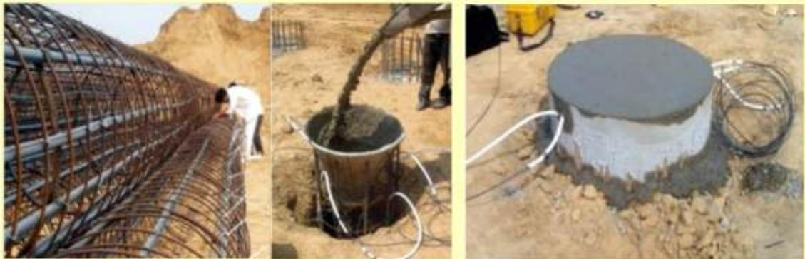
**Preparation of a pile for strain measurements Prepared pile with fiber cable**
